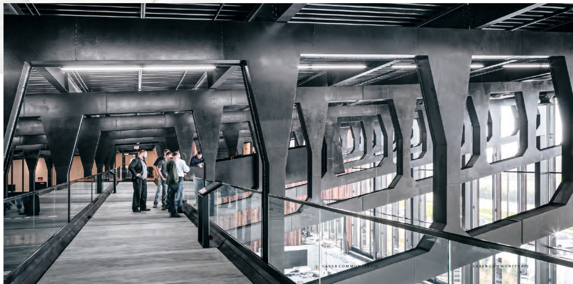
The roof of the production facility at the TRUMPF Smart Factory in Chicago is supported by eleven steel trusses, each made up of many individual pieces welded together.
